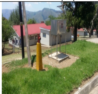
Figure 3-3: Fire water hydrant and hose reel
