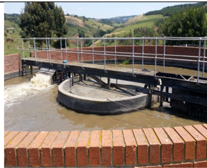
Figure 3-8: WWTW Settling tank
