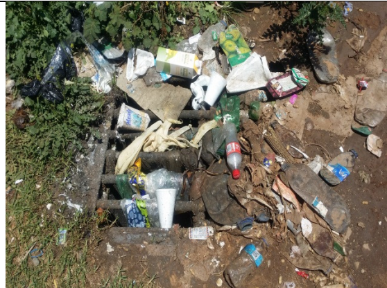
Figure 3-12: Blocked grid inlet
