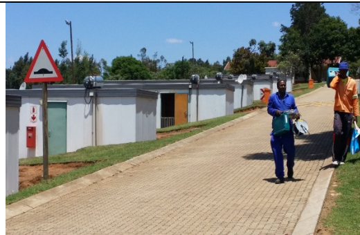
Figure 3-14: Kerbs forming a channel along the segmented block paving
