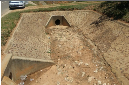
Figure 3-13: Grouted stone pitching with silt deposition
