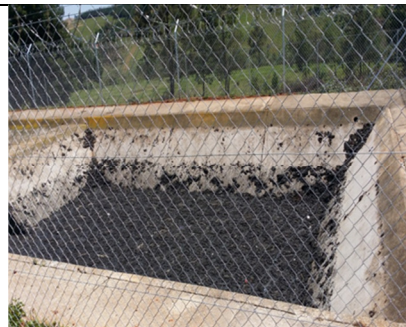
Figure 3-10: WWTW aerobic tank used as a drying bed
