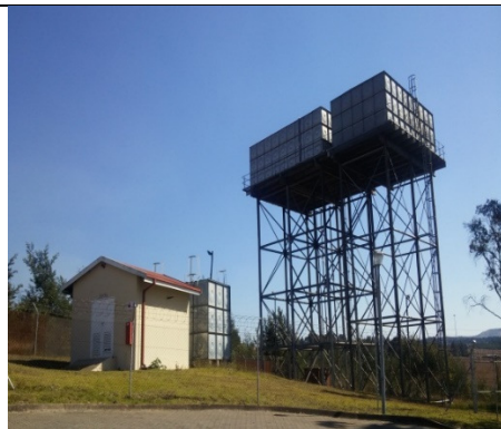
Figure 3-1: Two elevated potable water tanks, firewater tank and fire pump station
