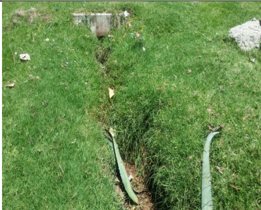
Figure 3-11: Earth channel overgrown with grass
