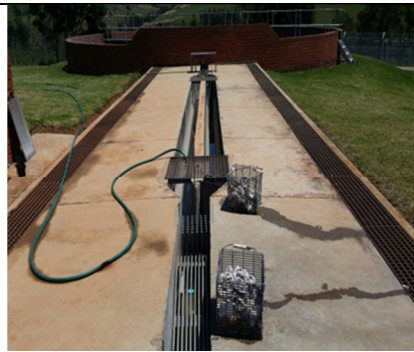
Figure 3-7: WWTW Inlet headworks
