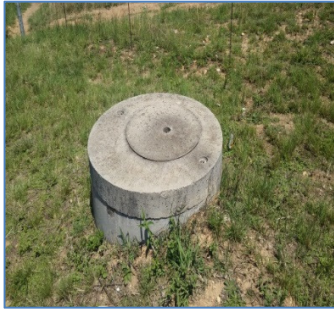
Figure 3-5: Non-overflowing manhole
